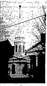
Up The steeple was elevated ento the Second Reformed Church last week. The unit is made of porcelain enameled from Columbia, South Carolina via truck and railroad. It weight 15,000 lbs., is 931/2 feet and cost more than \$17,000.
